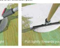
surface. Do not overwork the product by trying to spread it farther than it naturally wants to go. Remember to keep light pressure on the applicator. It is important to note that if there is Texture Coat build up on the Applicator blade, to clean it and re-wet the blade as you go. This keeps the blade
